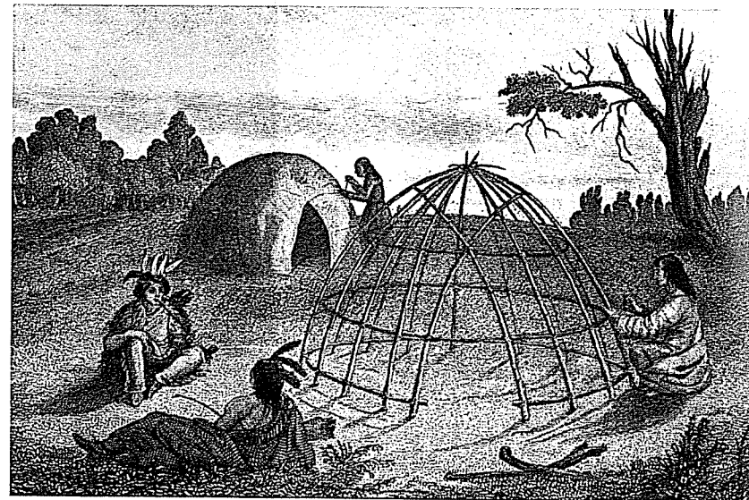
When the Algonquin moved, they would often take the wigwam's covering with them, but leave the poles behind. This way, they would not have to rebuild the frame when they returned to the area.
