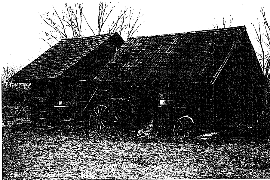
Father Pandosy's first building was a log chapel with living quarters above. The larger building beside it was a root cellar with walls of parallel logs built four inches apart and packed with earth to insulate the fruits and vegetables stored for the winter. | KELOWNA PUBLIC ARCHIVES 7075
